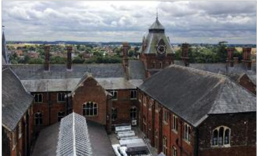
ABOVE: VIEW FROM THE COLLEGE CHIMNEY LOOKING SOUTH
